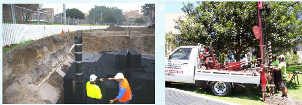
Photos: Installing the percolation tank under the Village Green at UNSW and drilling rig installing multi-level monitoring piezometers.
