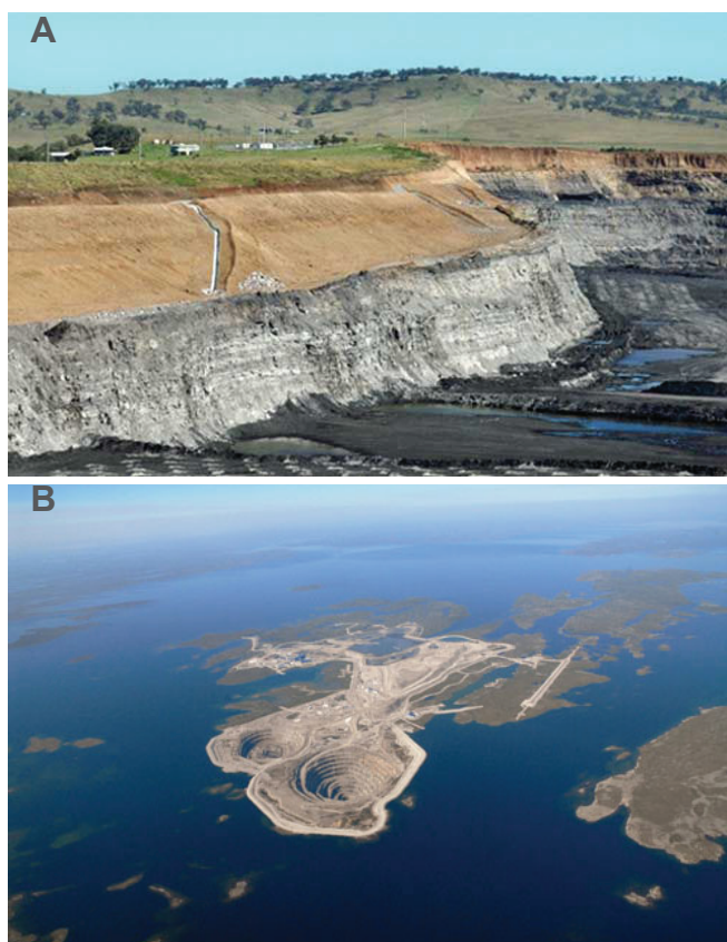
FIG 2 - Photographs showing (a) low permeability barrier (LPB) wall to limit seepage from an alluvial aquifer above coal in the Hunter Valley (Daracon, 2010); (b) LPB walls between an open pit diamond mine and a lake (Brunner and Schwank, 2003).
